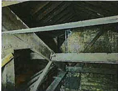
General view showing previous house wall
