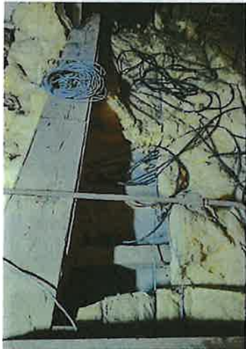
Polythene under Insulation
