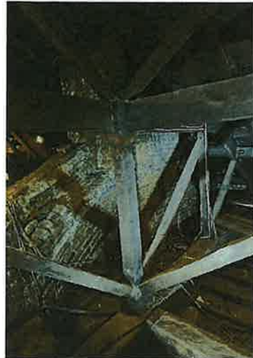
Second Former House Wall and Flues
